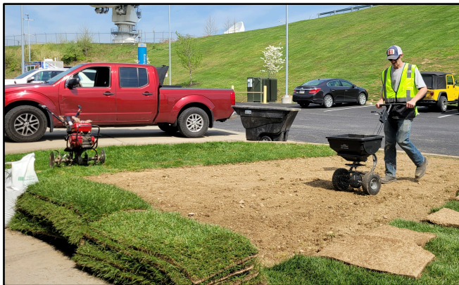
A student prepares a site for a sod installation.
