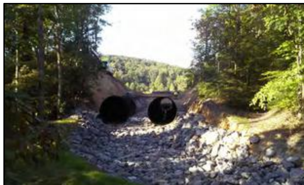
Two culverts installed on the Tibbs Run dam will create opportunities for new features at WVBG.
