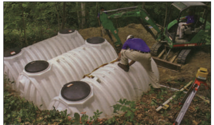
above: three 1,700 gallon tanks being installed for rainwater harvesting. photo by Robert Rivera
