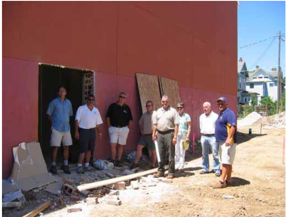
On June 11, 2008, WVNLA Board Members stand in the new doorway cut to provide access to the neighboring vacant lot from the Sojourners' Shelter Building. The lot will be landscaped as a gathering space for Shelter residents. From left to right: Treasurer Mark Springer; President Cary Levenson; Vice-President Brett Merritt; Past-President Norman Cole III; Bruce D. McClanahan of McClanahan Construction Company, Poca, WV, managing the project; Director Becky Morris; Director Bill Mills; and Director Tracy Cutlip.
